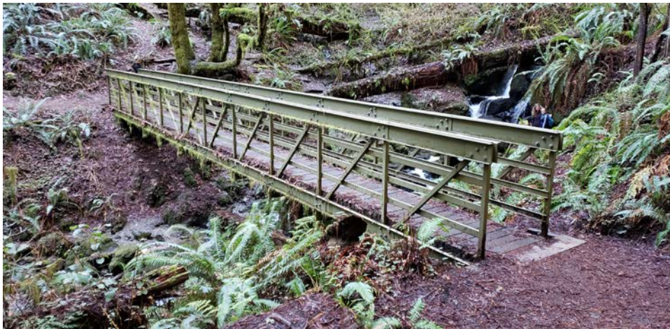
Photo 4-2: Fiberglass Bridge, Redwood National Park
