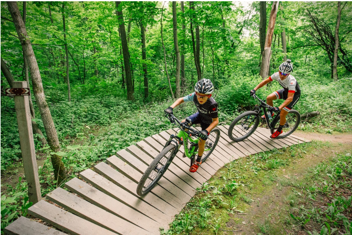
Figure 16. North Shore style wood feature.
