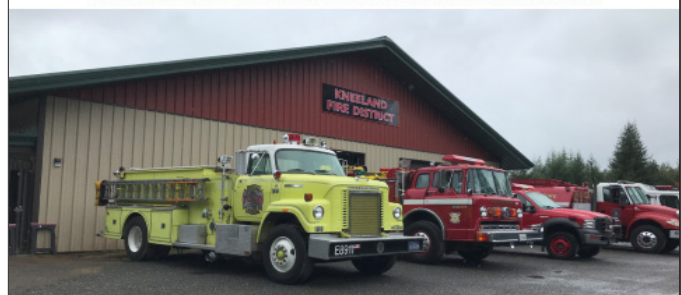
Measure Z Funded Kneeland Fire Station
