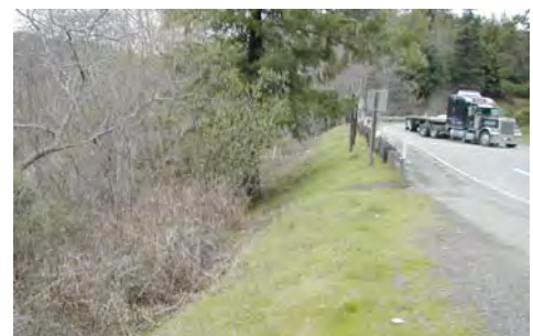
The trail would need to be located adjacent to and south of SR 299, perched above the Mad River.
