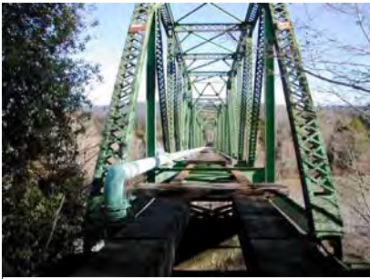
The A&M Mad River Bridge needs to be maintained because it also supports a HBMWD water line that serves Glendale, and Blue Lake.
