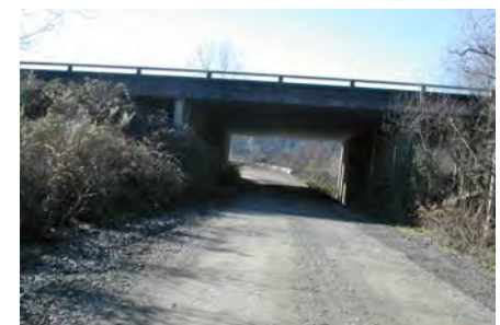
This private SR 299 undercrossing would be shared with industrial truck traffic in Glendale Alternatives D and E.
