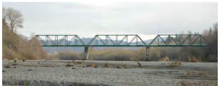
The 620-foot long Mad River bridge mostly consists of a steel truss superstructure much like that of the Hammond bridge.
