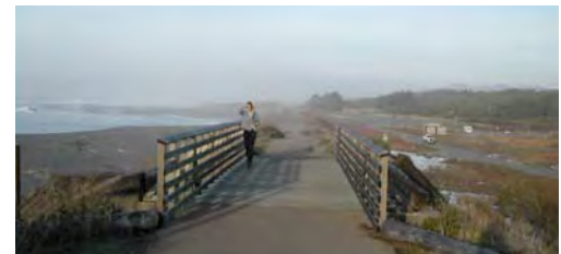
Wooden decking and railing on the McKerricker rail-trail in Mendocino County.
