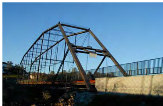
The historic Klamath River bridge was reinstalled for City of Folsom bikeway crossing at Lake Natoma. The retrofit included installation of the 54-inch high steel tubing fence for trail user safety.
