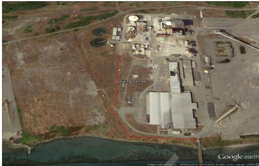
Figure 13 – Aerial Photo Showing Above Ground Plumbing Corridor
