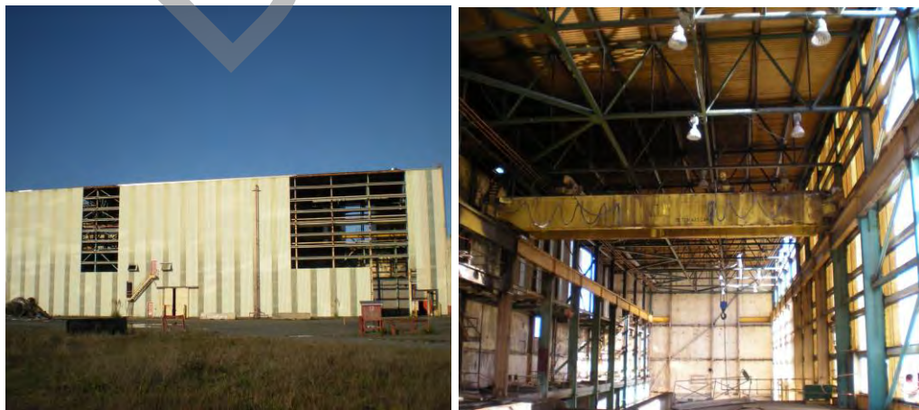
Figure 9 – Paper Machine Building – Outside South Side and Inside
