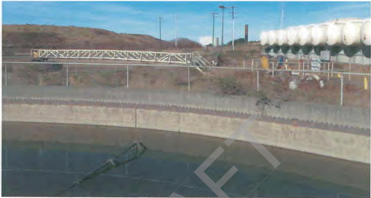
Figure 1. Humboldt Bay Municipal Water District Industrial Water Reservoir (white tank in distance) as viewed from the Freshwater Tissue Pulp Mill site water treatment plant.
