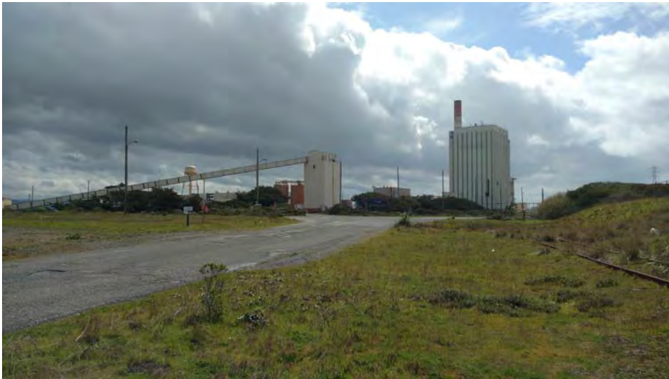
Photo B-4: Typical conditions within the project area. Samoa effluent pipeline proposed to be placed between Vance Avenue (left) and the railroad. Photo taken 3/23/2017.
