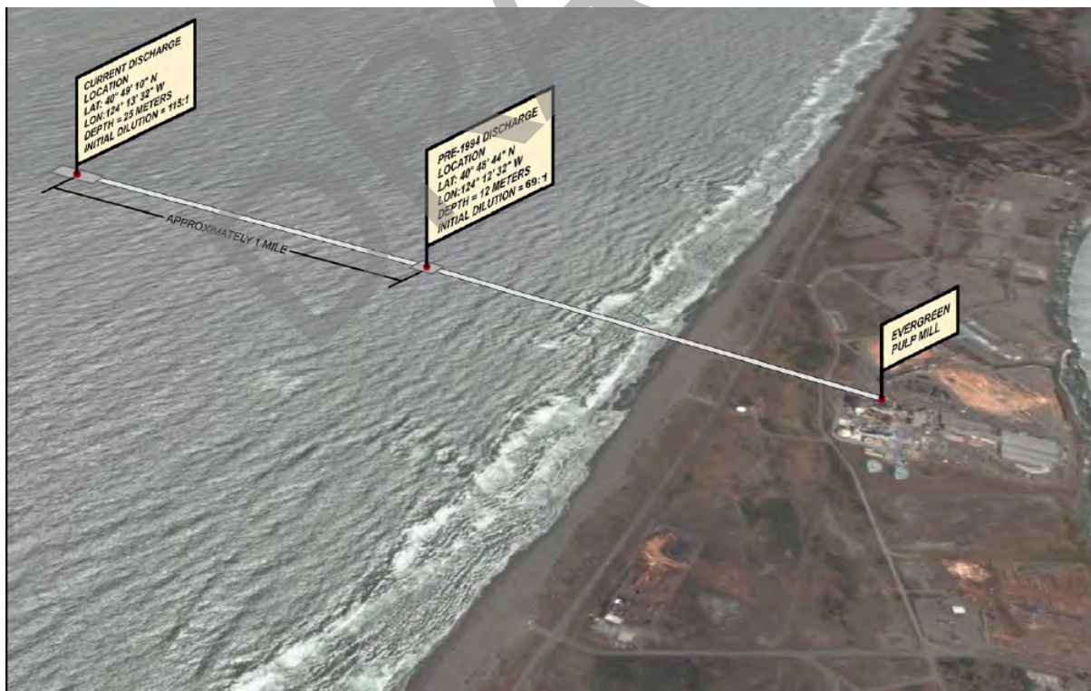
Figure 2. A picture of the location of the RMT II ocean outfall and diffuser.
