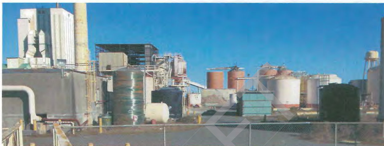
Figure 3. Freshwater Tissue Pump Mill site including numerous spent liquor tanks.
