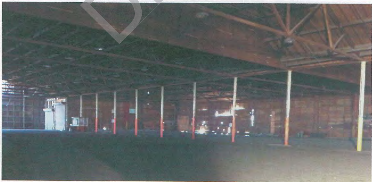
Figure 6. Interior of Warehouse #2.
