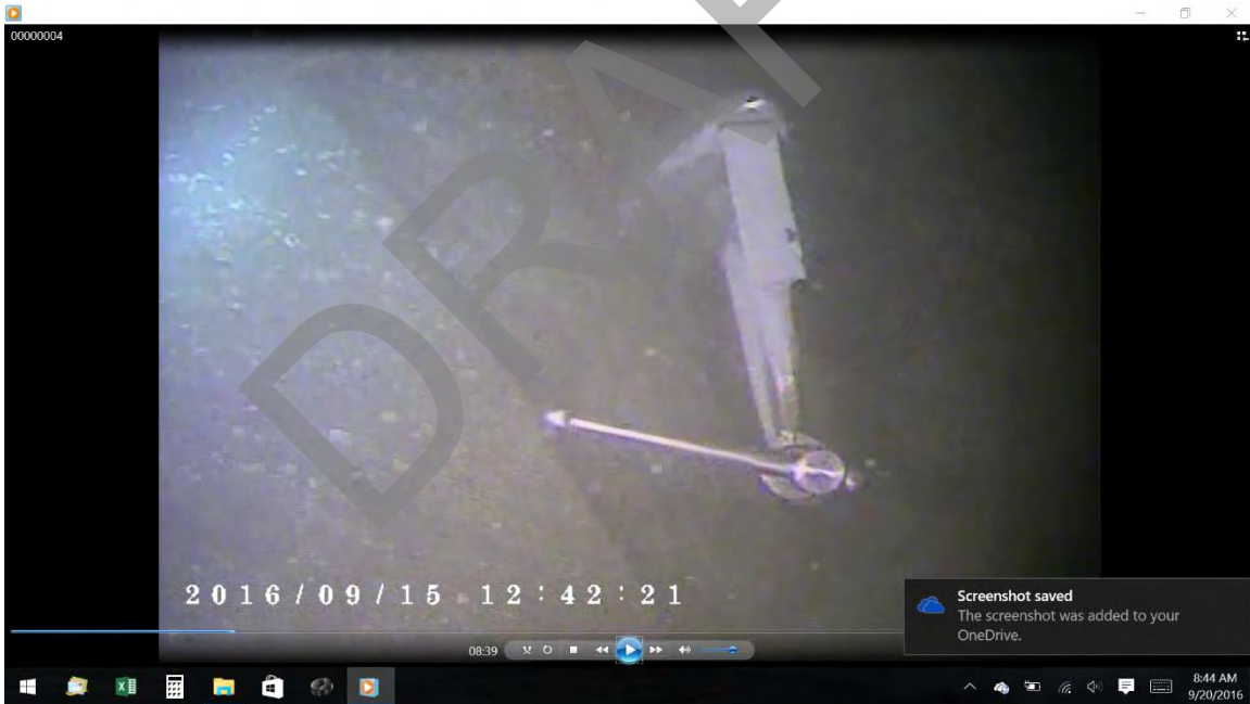
Figure 4 Zinc anode attached with C-clamp to depleted ankle bracelet quadrant
