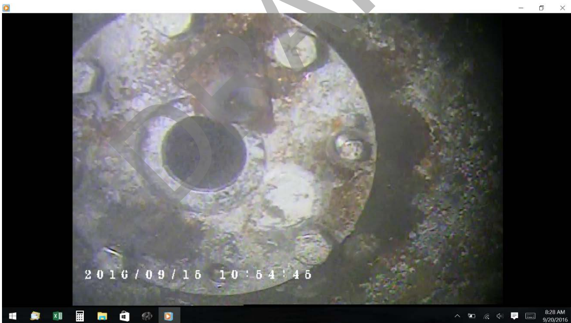
Figure 2 Assembling diffuser port after internal jetting.
