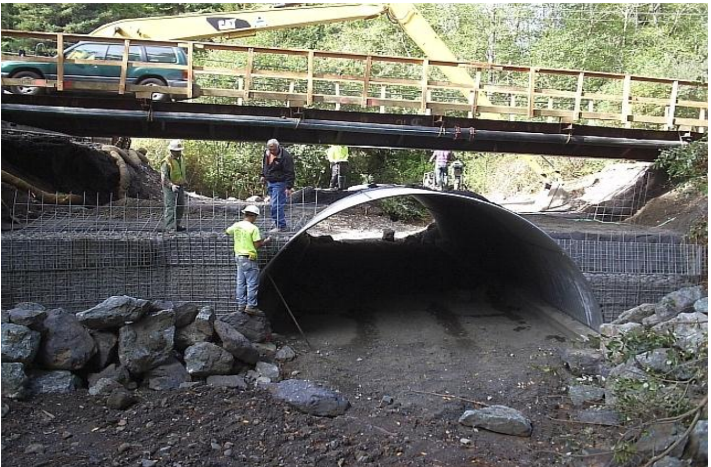
Public Work's fish-friendly culvert replacement project at Grassy Creek
