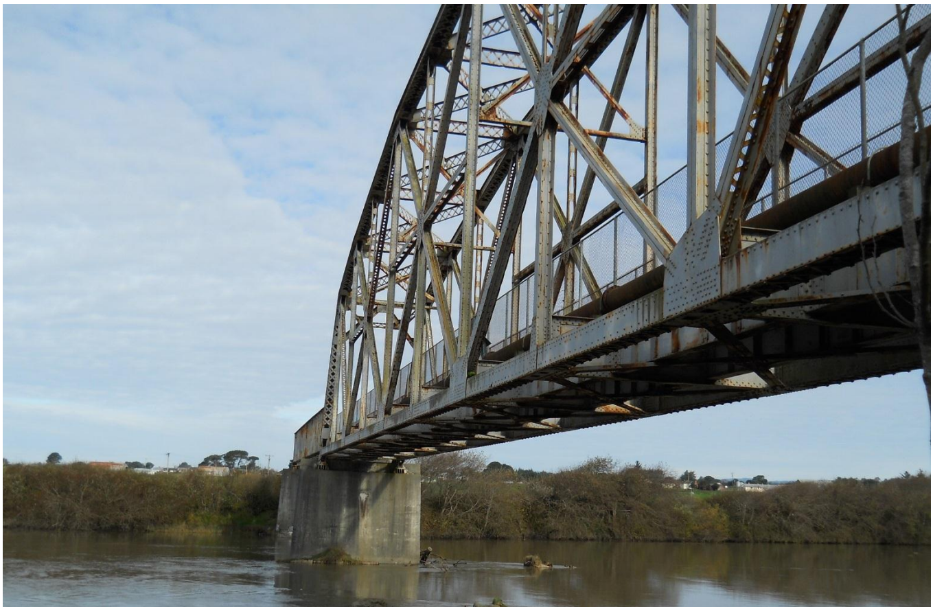
Hammond Trail Bridge over the Mad River
