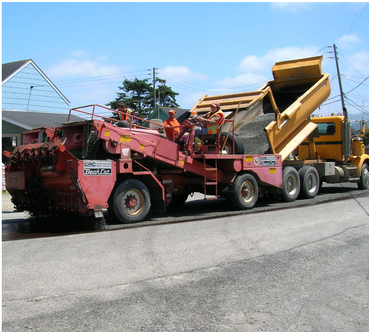
Road crew staff chip sealing a County road
