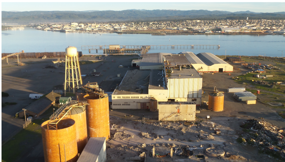
View of Terminal 2 and buildings on Samoa Peninsula
