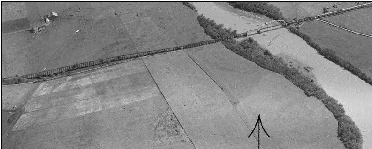
Illustration 6. Aerial photo from 1953 showing bridge and trestle sections on each side. This view is looking southeast. 30
