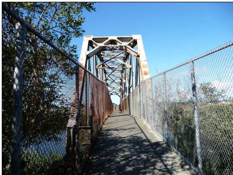
Photograph 3: Span 4, camera facing north, September 25, 2013.
