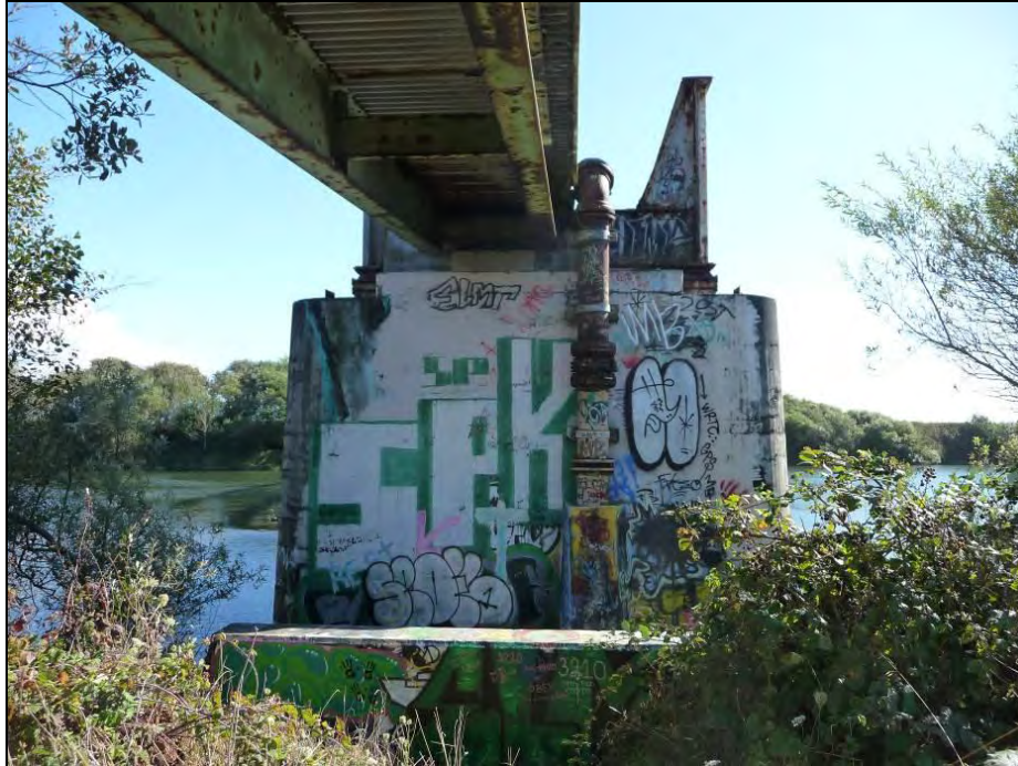
Photograph 16: Intersection of Span 2 and Span 3, camera facing south, September 25, 2013.
