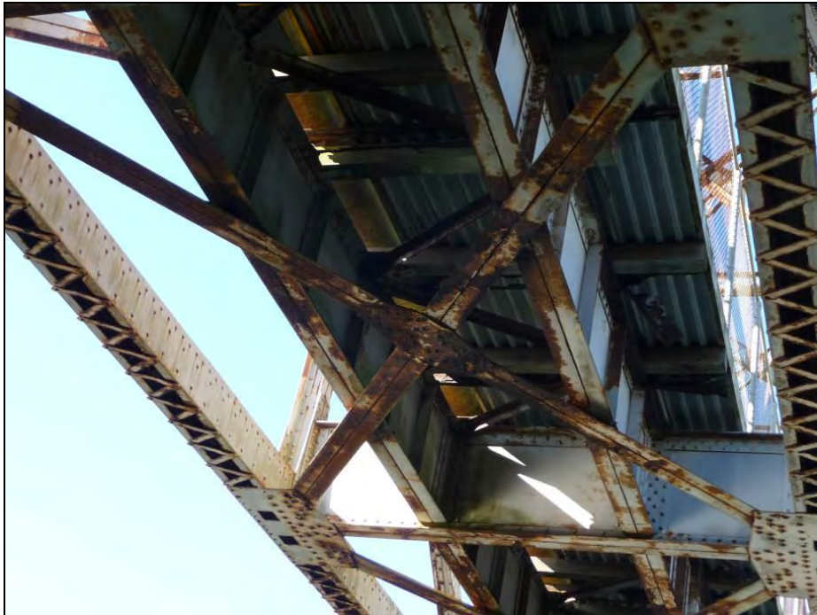
Photograph 6: Span 4 below deck, camera facing northwest, September 25, 2013.
