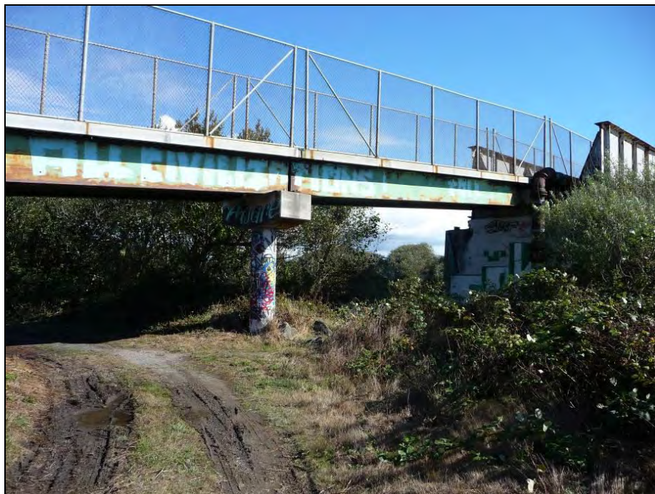
Photograph 13: Span 1 and Span 2 camera facing southeast, September 25, 2013.
