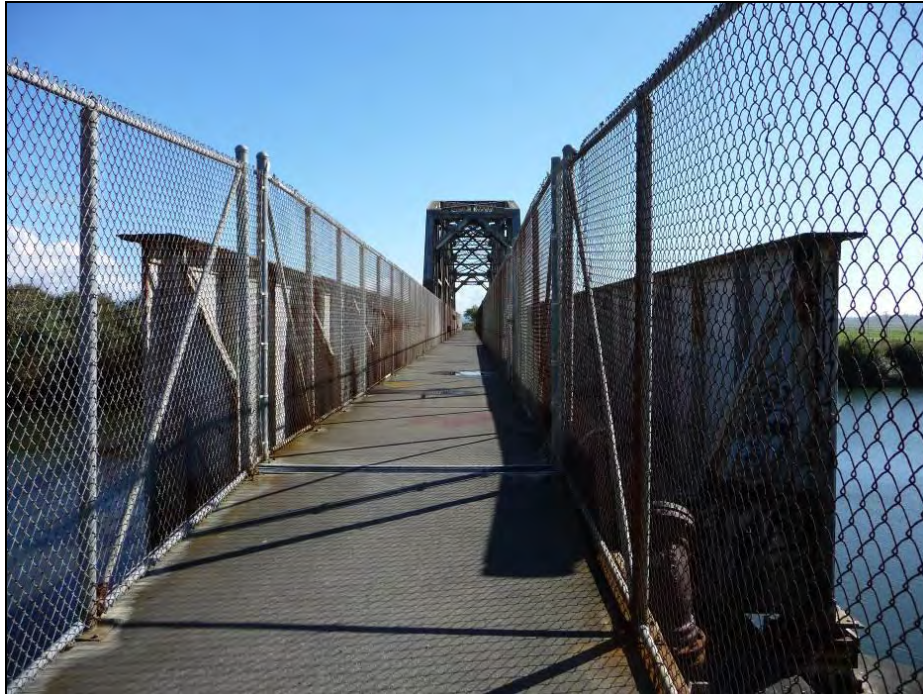
Photograph 10: Span 3, camera facing south, September 25, 2013.
