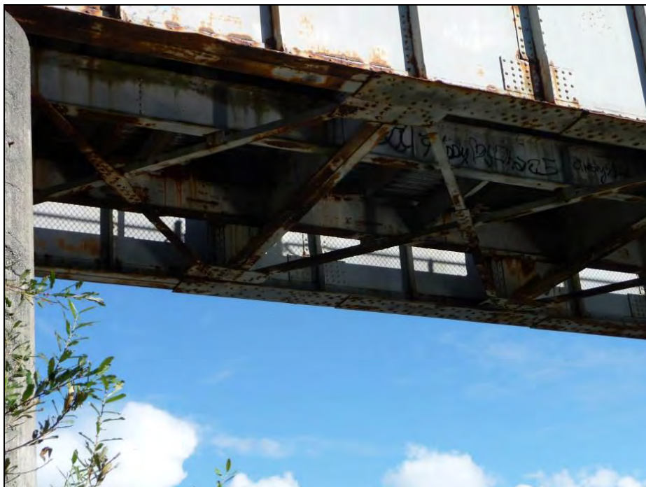
Photograph 11: Span 3 below deck, camera facing east, September 25, 2013.
