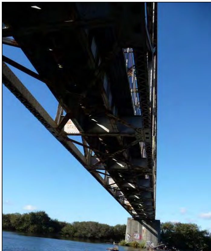
Photograph 7: Span 4, camera facing north, September 25, 2013.
