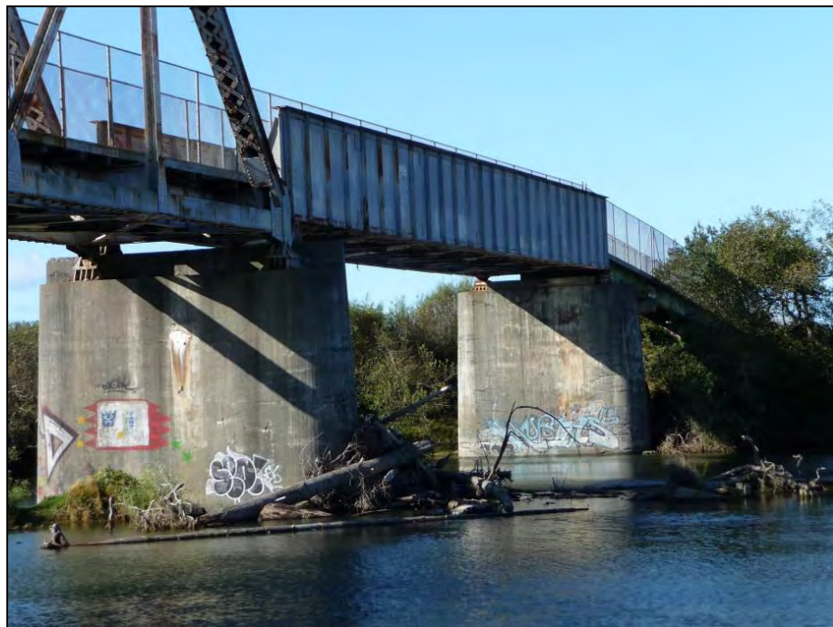
Photograph 9: Span 3, camera facing northwest, September 25, 2013.
