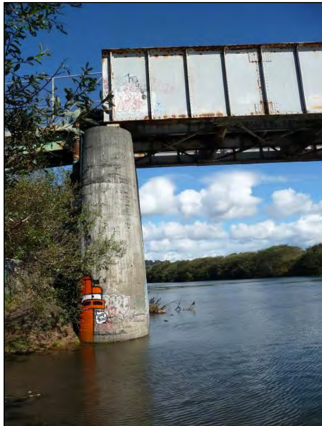
Photograph 12: Intersection of Span 2 and Span 3 camera facing east, September 25, 2013.
