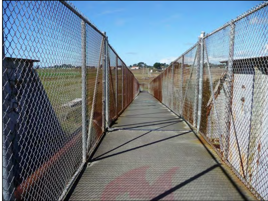
Photograph 14: Span 1 and Span 2 camera facing north, September 25, 2013.
