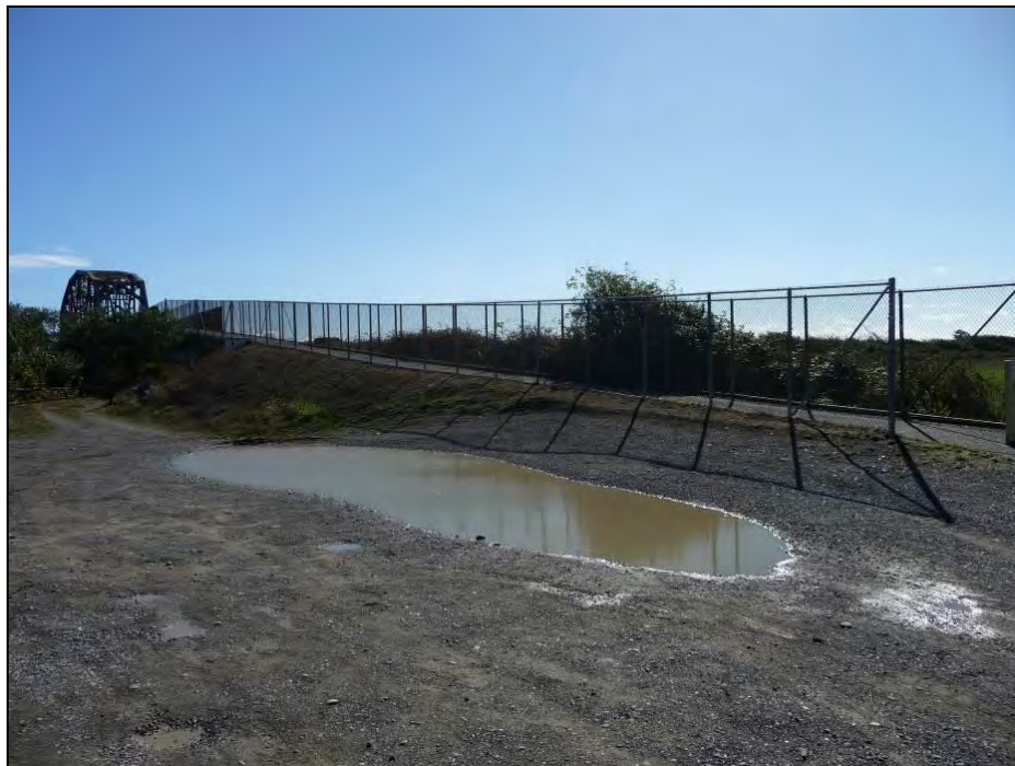
Photograph 17: Bridge approach from north, camera facing southwest, September 25, 2013.
