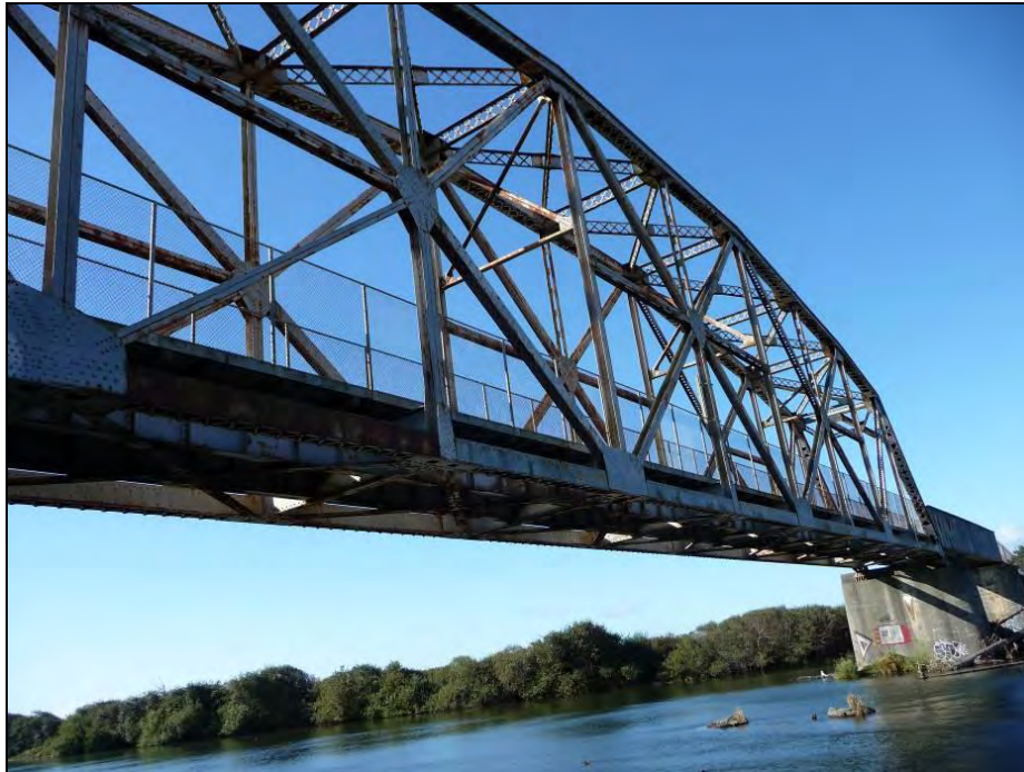
Photograph 2: Span 4, camera facing northwest, September 25, 2013.
