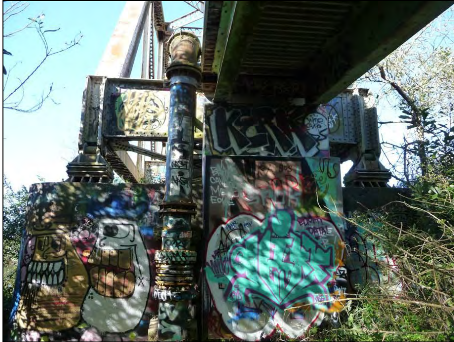
Photograph 8: Intersection of Span 4 and Span 5, camera facing north, September 25, 2013.
