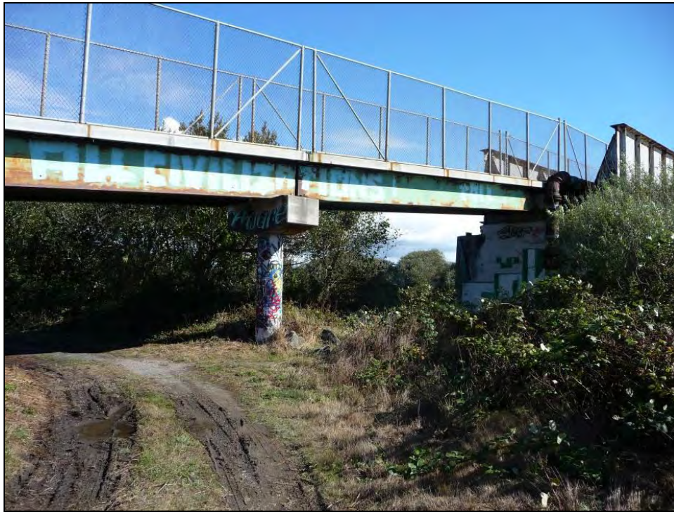
Photograph 3. North bridge approach built in 1983, camera facing southeast, September 25, 2013.
