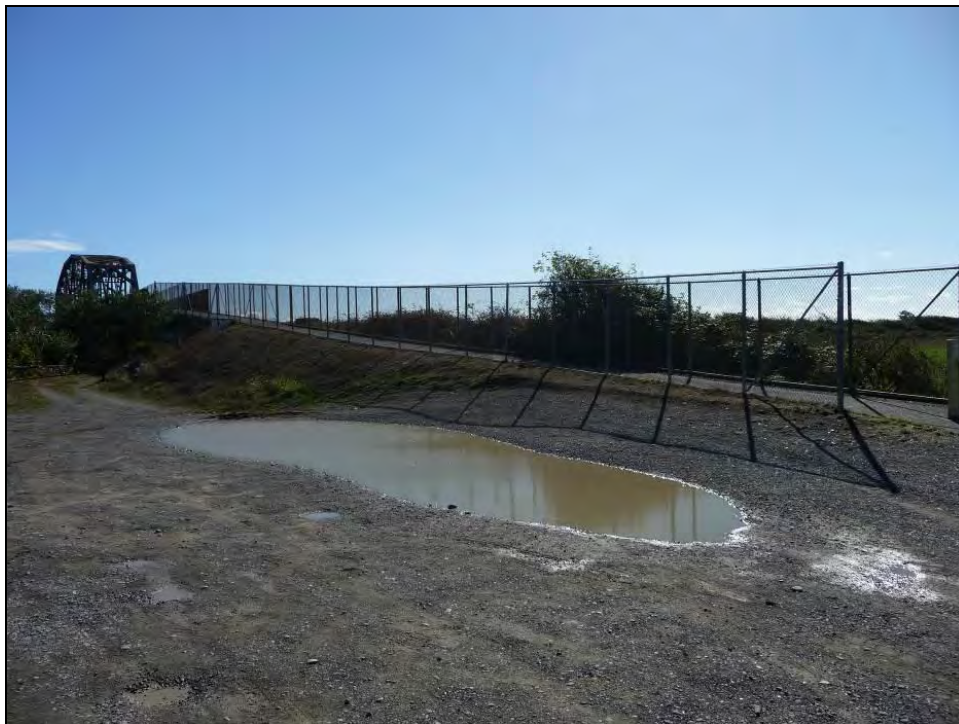
Photograph 4. North bridge approach built in 1983, camera facing southwest, September 25, 2013.
