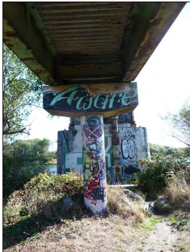
Photograph 15: Span 1 and Span 2 below deck, camera facing south, September 25, 2013.
